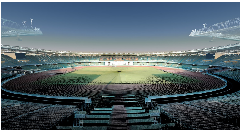
Sports stadium in Abu Dhabi. Point cloud processed using Pointools Edit
